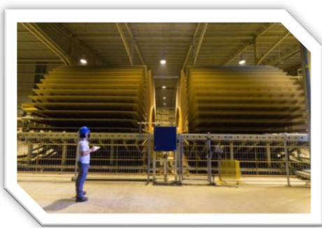
COOLING STACKING & HANDLING SYSTEM
