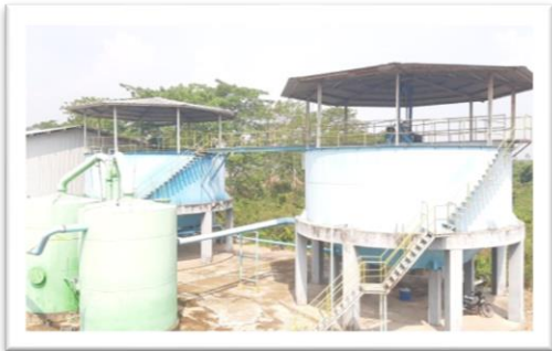
WATER TREATMENT PLANT
